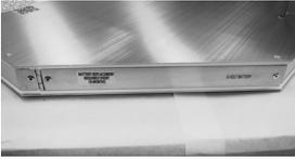
2. Use a razor knife and cut one slice through each bead of caulk. DO NOT remove caulk.
