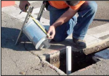
*Mounting Jig Attached to Base Can*
